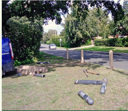
Bollard replacement at Silkmore Lane
