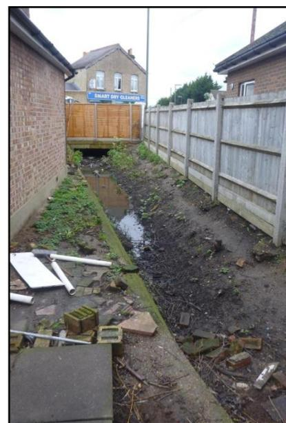
*Figure 3-A ditch in need of maintenance which includes removing vegetation, silt and other debris*
