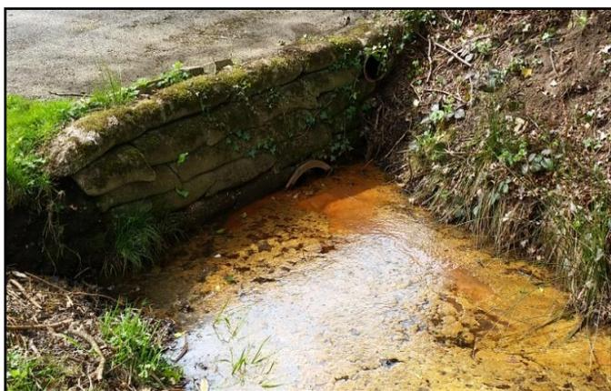
*Figure 4-A ditch where silt has built up over the opening of a pipe inlet*
