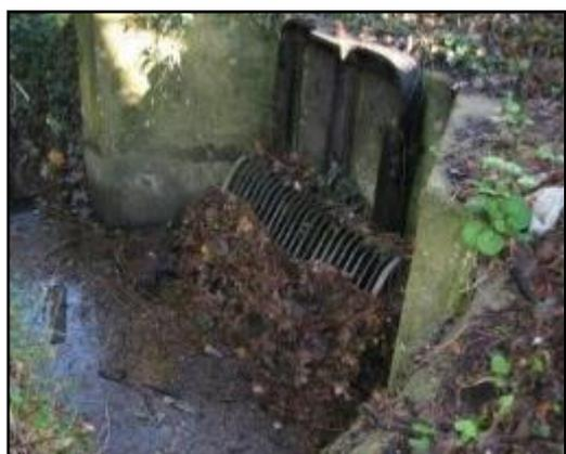
*Figure 6-A trashscreen with a build-up of leaf litter and other debris causing an obstruction to the flow of water*
