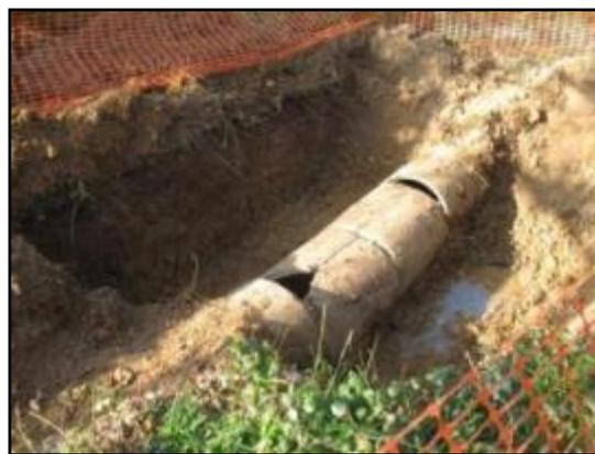
*Figure 5-A damaged culvert requiring repair*
